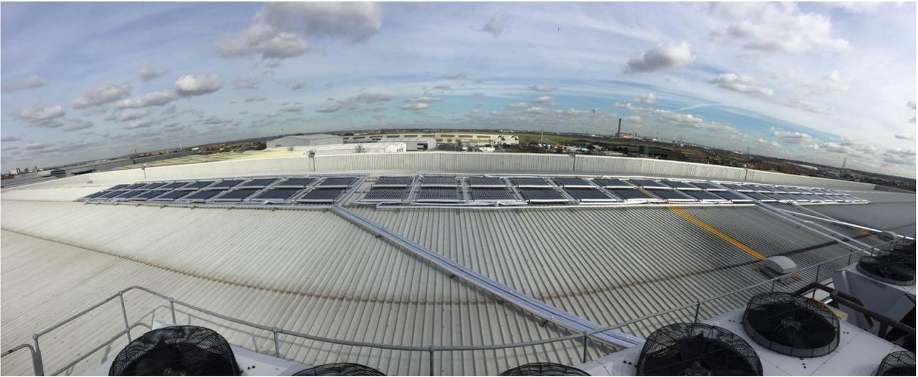
Image 2: the solar thermal collectors installed in parallel on the roof of the Chingford fruit facility. *Source SCE picture gallery*
